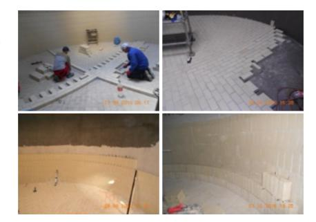
All applied systems are composed of multiple layers of linings (resin layers, reinforced fiber glass layers), rubber membranes, acid-proof bricks (carbon bricks, ceramic bricks), special acid proof mortars and epoxy coatings. Materials recommended and produce by our partner Tip Top Oberflächenschutz Elbe GmbH are distinguished both by excellent chemical resistance which provides corrosion protection and abrasion resistance for wear protection.
